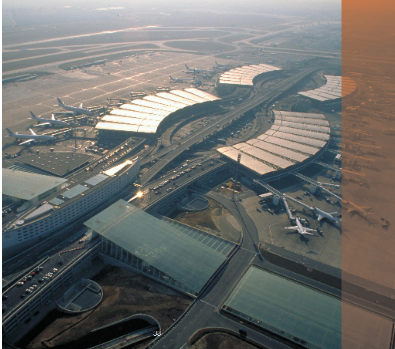
Aerial view of the terminals 2A, 2B, 2C and 2D and of the Paris-CDG 2 train station
